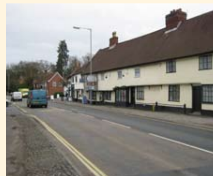
Building opposite Swan Lane. Dates from c16 and was originally 2 houses.
