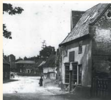
View along The Street looking north - late c19
