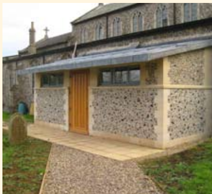
New extension at St Mary's Church
