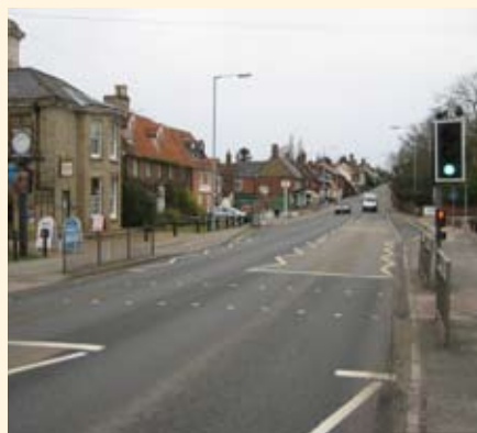
View west side of the street looking north from opposite the junction with Swan Lane
