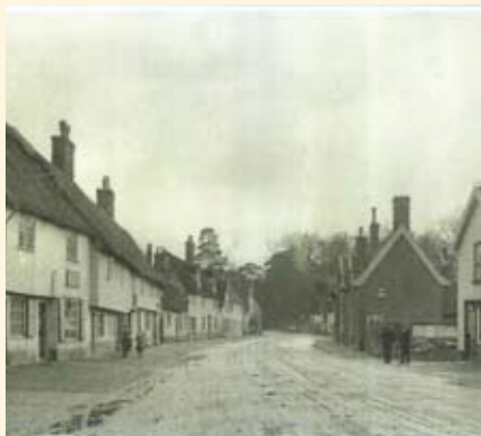
View south along the Ipswich Road 1908
