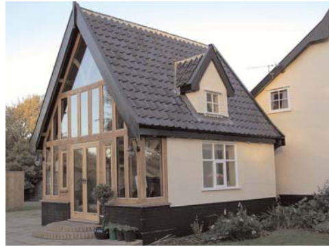
Extension to Existing Building Category Elm Tree Farm, Tivetshall St Margaret Paul Goddard, Architect
