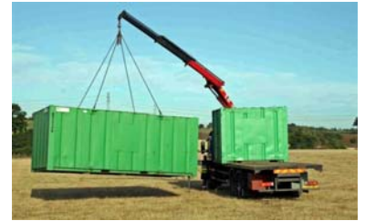
Day 2 The first of the three deliveries from our wonderful sponsors May Gurney and A Plant arrive. These containers were closely followed by all the bright shiny brand new equipment.
