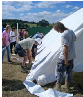
Day 4 Turf stripping continues with a welcome break when all bodies were summoned to help get the marquee erected.
